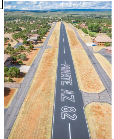
AZ82 Runway after crack seal and seal coating.
